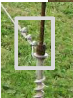
Cable clamps for guy-wire's loop around PE26
