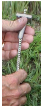
Thread Quickvise onto the cable and seat it into hole in the stud
