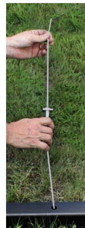
Thread Quickvise onto the cable and seat it into hole in the stud
