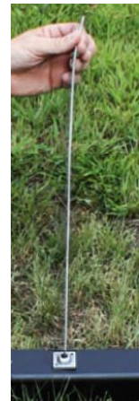
Pull cable to tension it, securing stud to the ground
